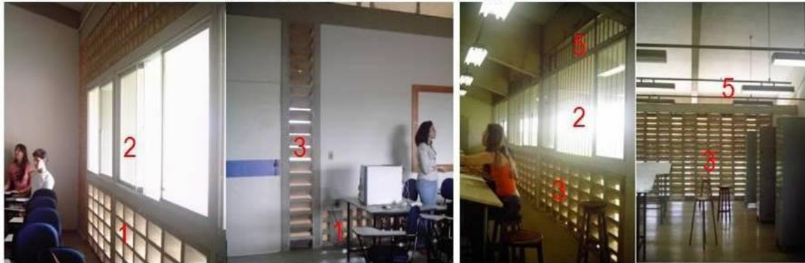
1: Perforated blocks 2: Sliding windows 3: Venetians (concrete) 4: Area for ventilation above the window 5: Open area for ventilation.
