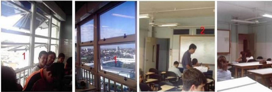
1: Sash windows 2: Venetians (iron).
