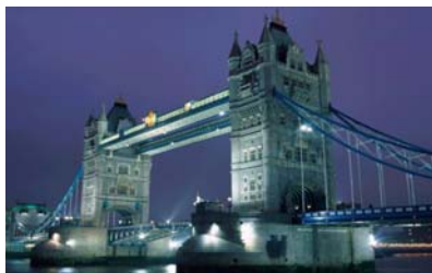
Figura 2.2 – Tower Bridge ( http://qualitywallpapers.x-istence.com/Nature , 12/12/2005)
