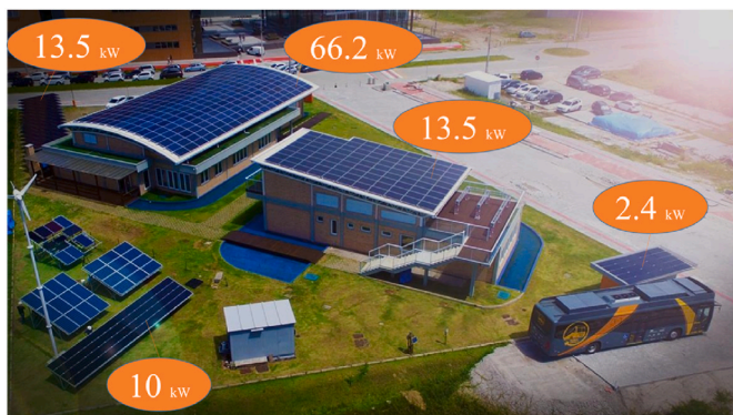
Fig. 4. The UFSC Solar Energy Research Laboratory's existing solar PV generators.
