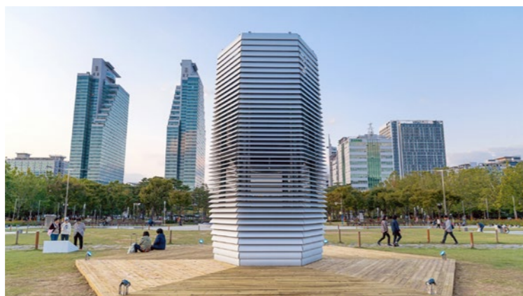
Figura 1: Smog Free Tower. Fonte: https://www.studio Roosegaard.net/project/smog-free-tower
