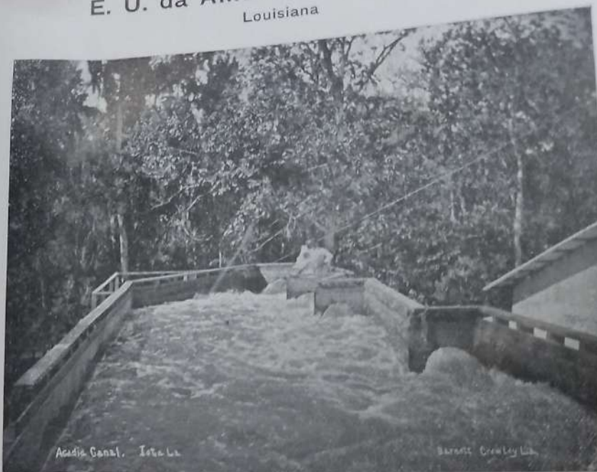
Descarga das bombas no canal principal
