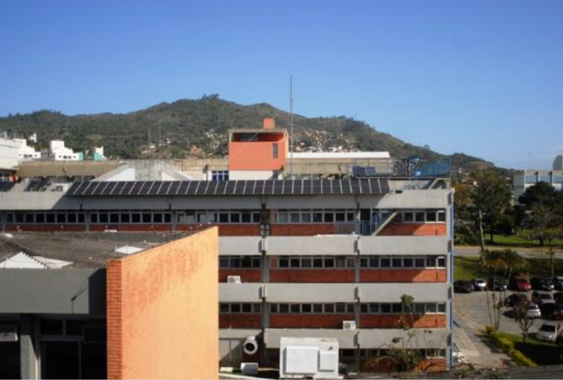
Figure 7 – Mechanical Engineering building's PV system.
