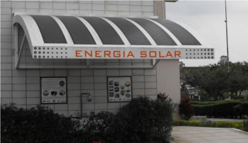
Figure 10 – Culture and Events Center curved rooftop PV system.
