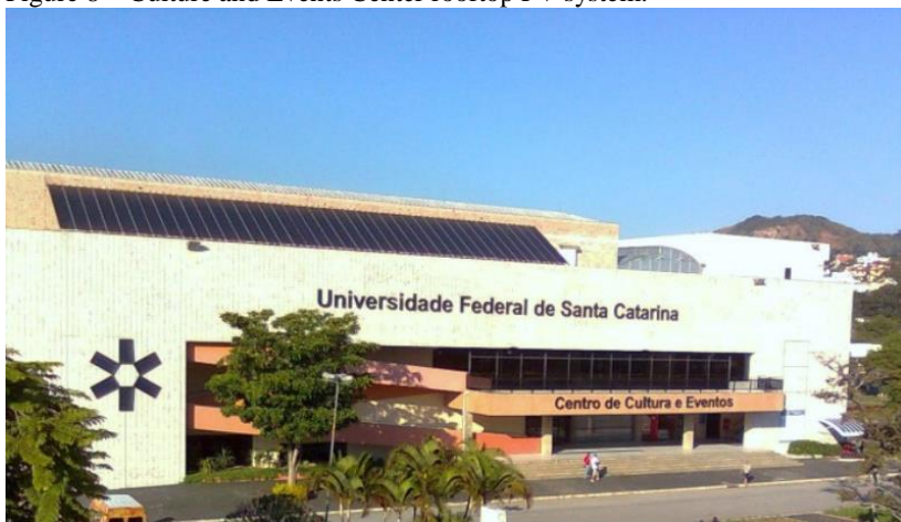
Figure 8 – Culture and Events Center rooftop PV system.
