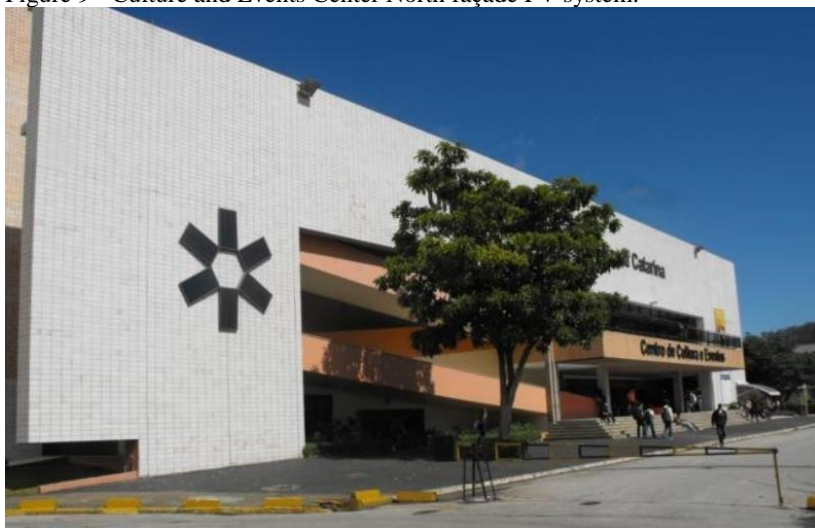
Figure 9 - Culture and Events Center North façade PV system.
