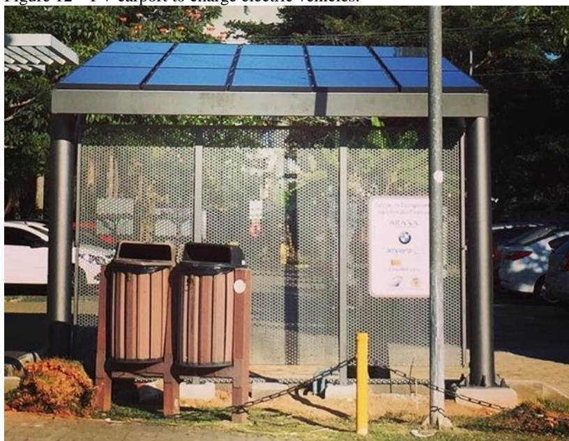
Figure 12 – PV carport to charge electric vehicles.
