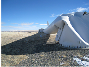
(a) Wind turbine collapse failure under extreme wind
