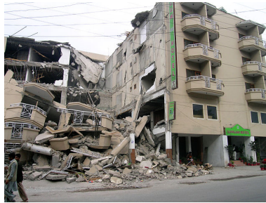
(b) Building collapse under earthquake
