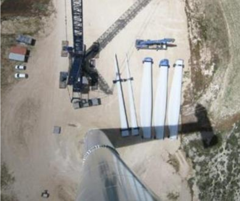
Figure 2.9 – Blade segments delivered to a wind farm await assembly. (Source: Gamesa [26])
