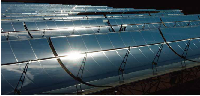
Figure 18: SkyTrough parabolic trough collectors.
