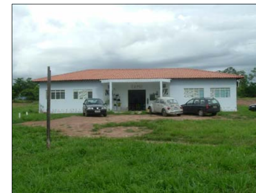
Figura 10: Vista Principal (V1)
