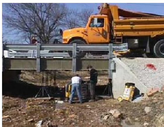
FIGURA 2.31 – St. Francis Street Bridge , instalada no Missouri. Fonte: NYSTROM et al. (2003).
