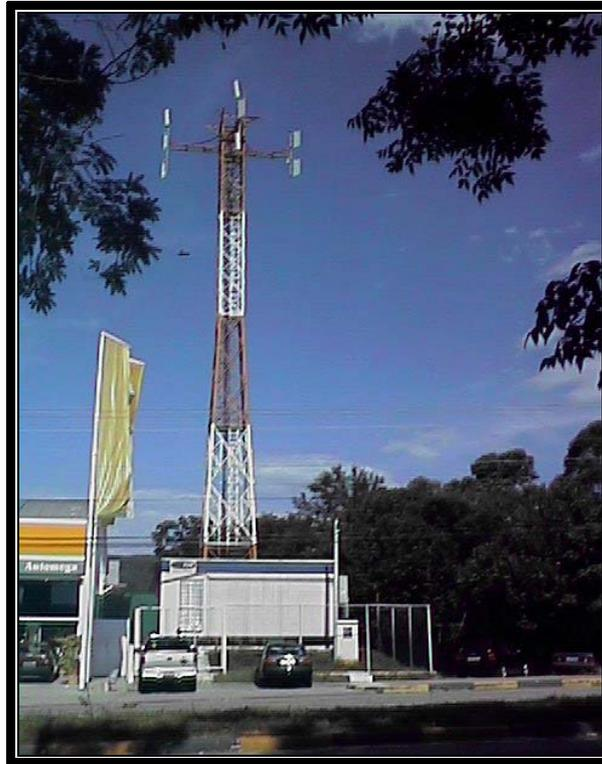
**FIGURA 1.1** – A torre, antenas e o container
