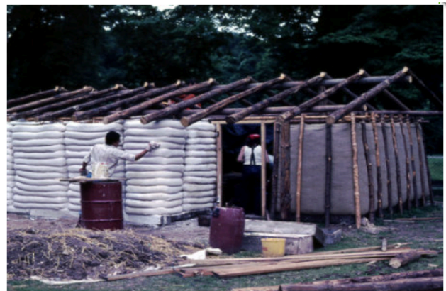
Figura 10 e 11: Earthquake resistant sandbag structure, Guatemala 1978. Fonte: Gernot Minke (2024) .
