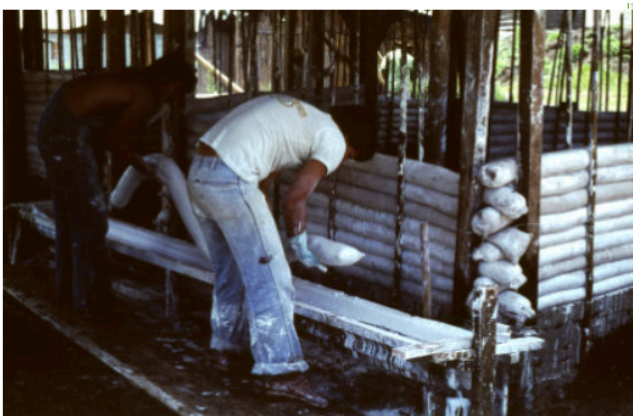
Figura 10 e 11: Earthquake resistant sandbag structure, Guatemala 1978. Fonte: Gernot Minke (2024) .
