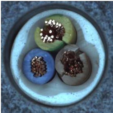
(c) Defected cable: cut inner insulation.
