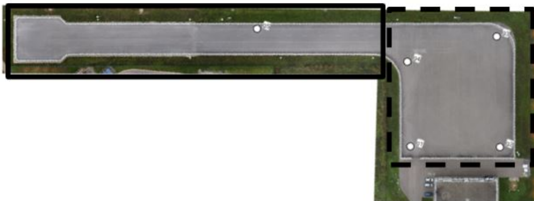
Figure 17 – CARISSMA outdoor test facilities, top view
