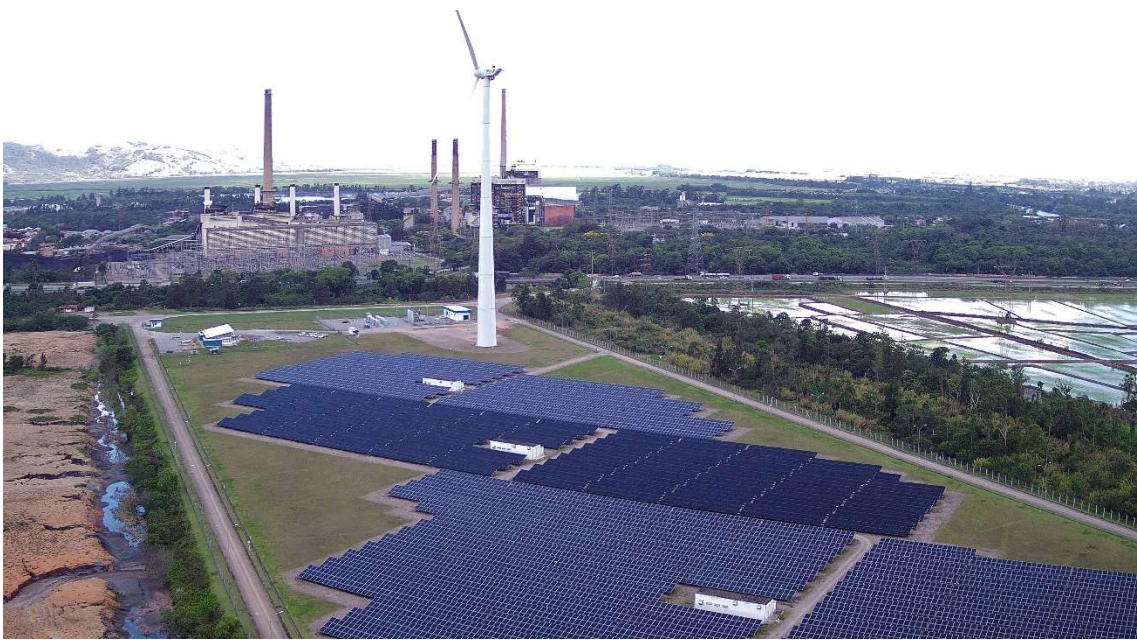
Figure 4-5 - The 3 MW R&D utility-scale PV power plant in the South of Brazil which was used as Test Case #1 to validate the method proposed here.
