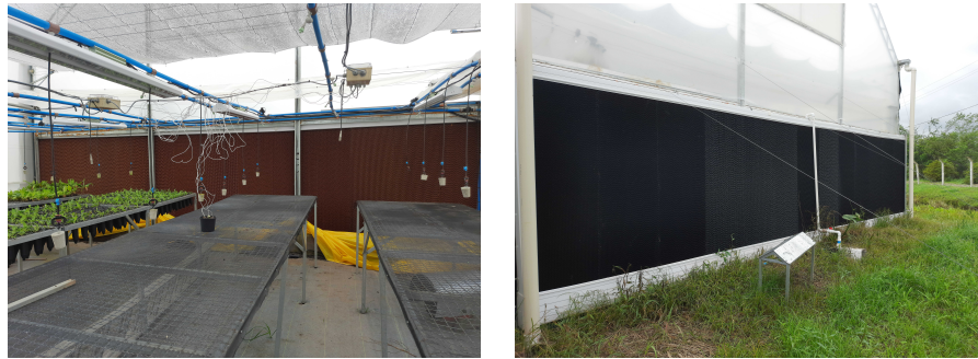
Figure 3: Humid Wall inside view at left and outside view at right
