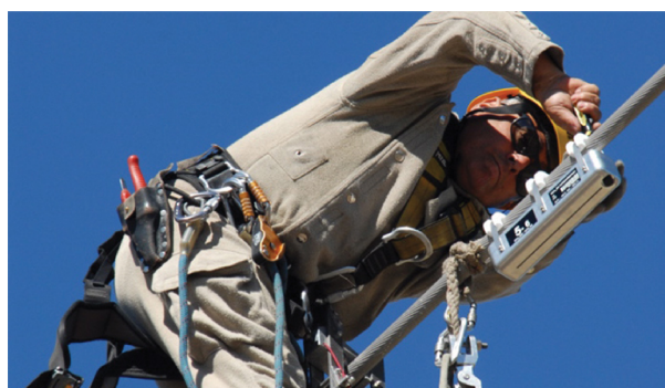
Figure 2.10 – EMO system live-line installation.
