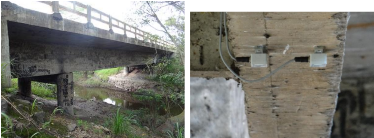
(a) Lateral view of the bridge
