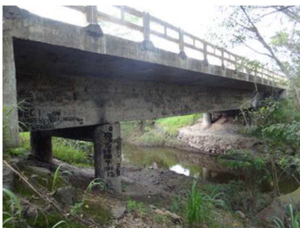
(a) Lateral view of the bridge
