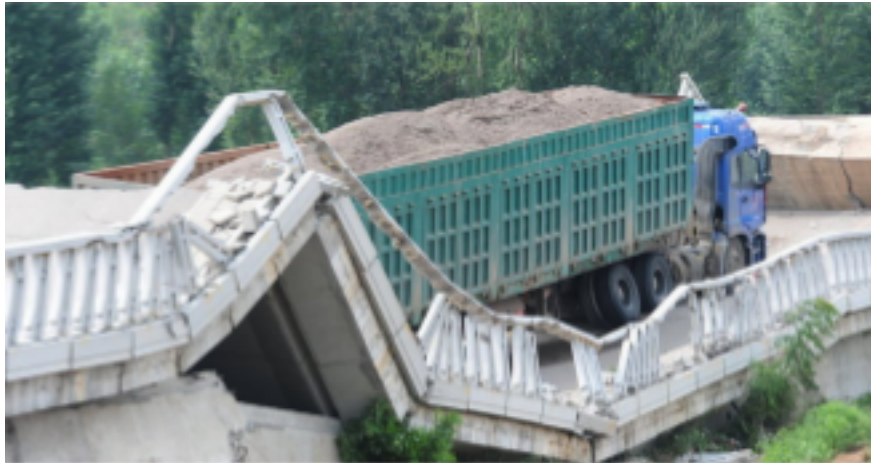
Figure 2 – Bridge collapse due to overloaded vehicle
