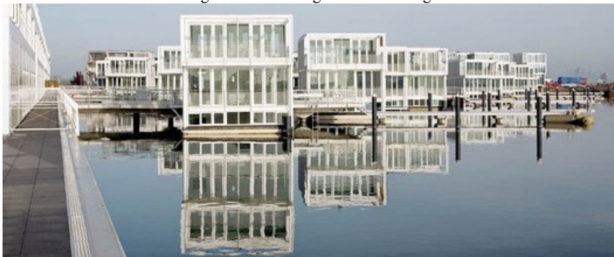
Figura 29 – Floating Houses – IJburg.
