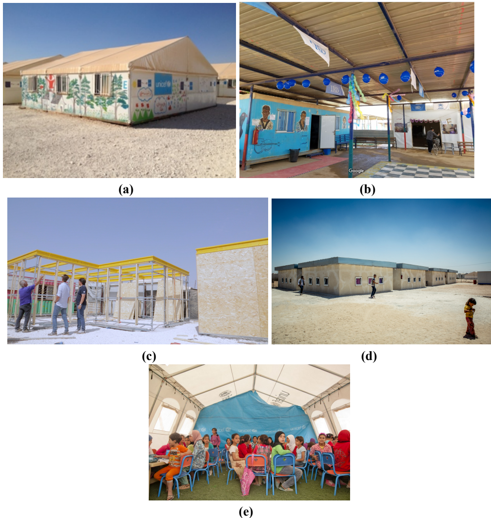
Figura 6: (a) (b) (c) (d). Escolas.(f) centro educacional Fonte: Disponível em: http://learning-reimagined.com/zaatari-refugee-camp-jordan/ , Google Maps (2021), https://www.dezeen.com/2017/07/20/building-peace-foundation-school-syrian-refugee-camp-zaatari-cameron-sinclair-architecture/ , https://learningspacealive2015.wordpress.com/future-learning-space-3/ . Acesso em: 27 jul. 2021.
