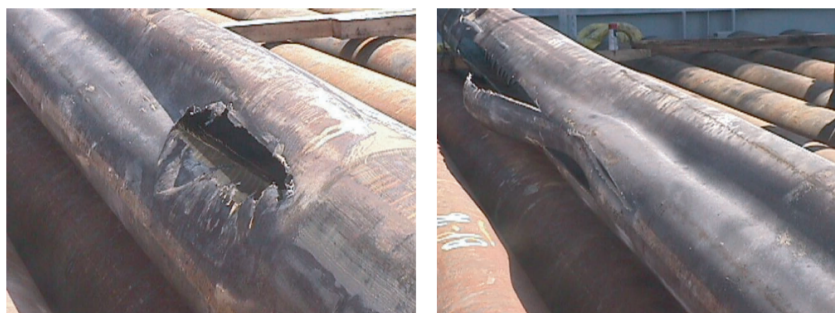
Figure 4 – Failure of the 16” casing in the Pompano A-31 well.
