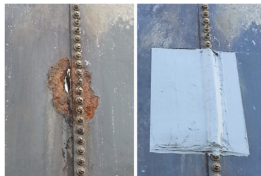
(b) Tank repair (BIG, 2021).
