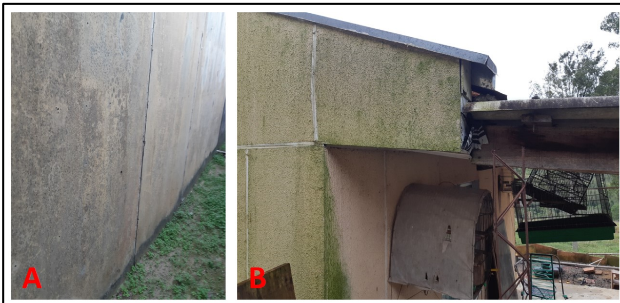
Figura 185 - Manchas causadas por microrganismos nas fachadas das HIS 2 (A) e HIS 9 (B).
