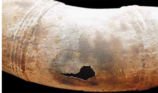
Figure 54: Failure due to erosion–corrosion in the elbow section (BHARDWAJ, 2020).
