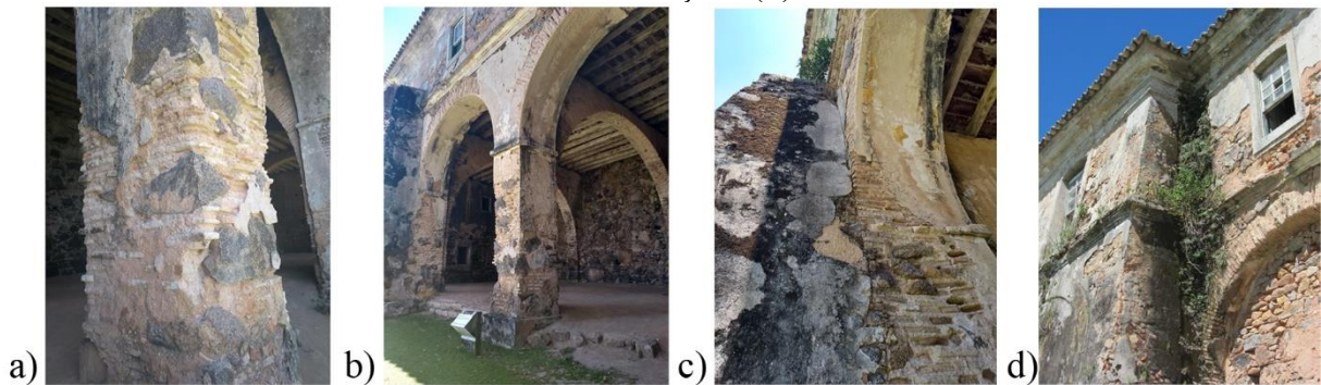
Figure 92 - Damages in the column of the 4th axis of the structure (a, b), connection between column and buttresses (c) and connection of the central slope-shaped masonry with the main façade (d).
