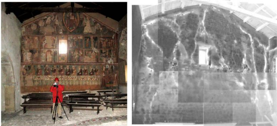
Figure 8 - Endangered fresco by an earthquake: picture and thermographic detection of delaminations and structural cracks.
