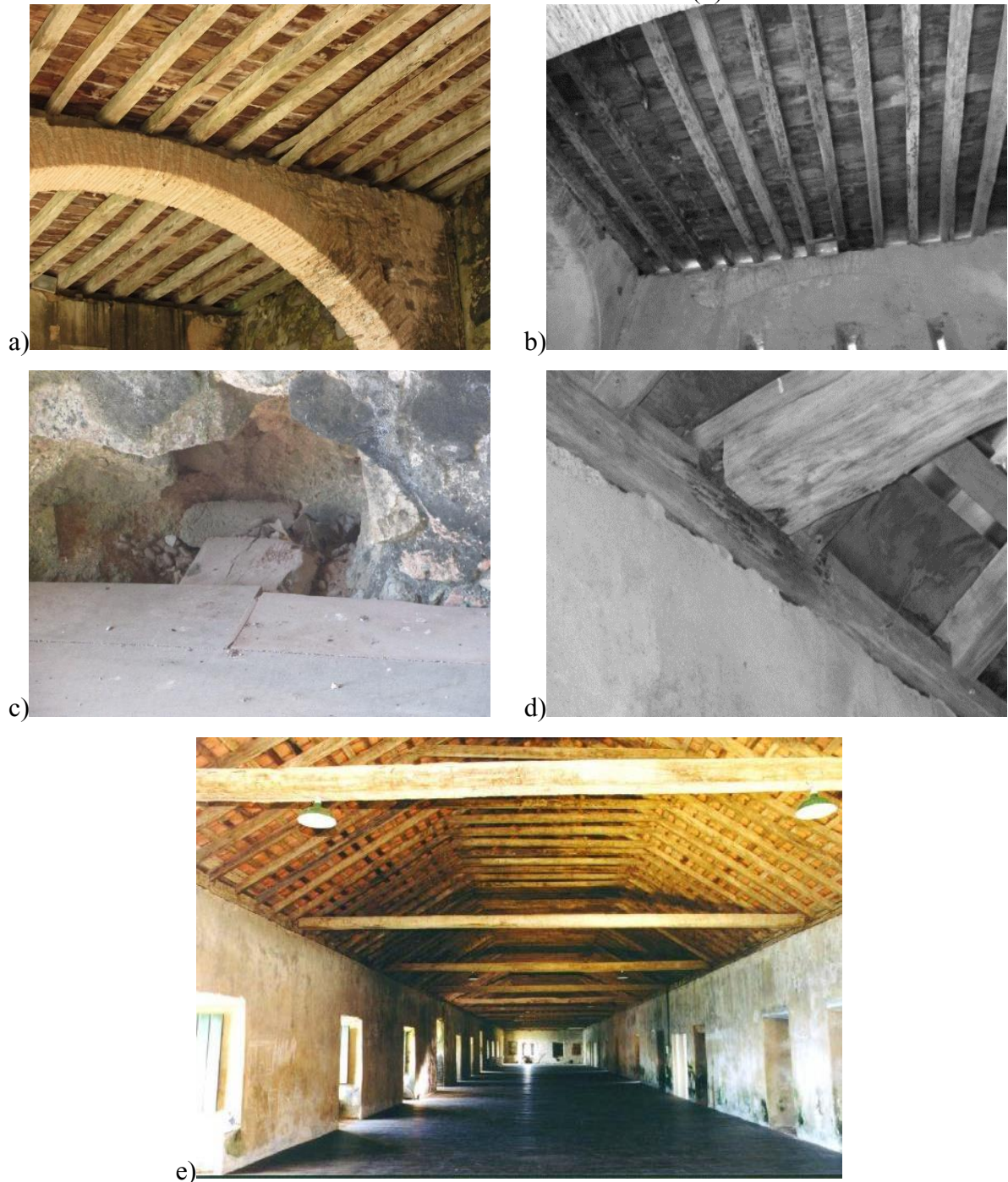
Figure 80 - Current state of the wooden slab elements (a, b), supports of the wooden slab (c) and the wooden tie-beams of the roof (d).
