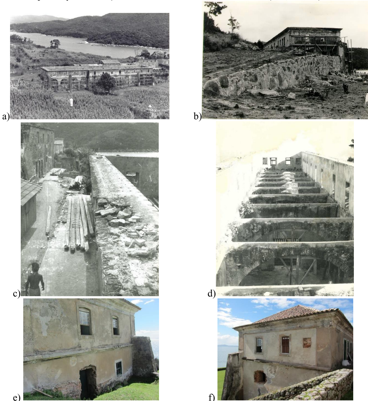
Figure 76 - Quartel das Tropas in the 1970s structural interventions (a, b, c, and d). Lateral partially buried façades in three sides of the construction (b, c, e and f).
