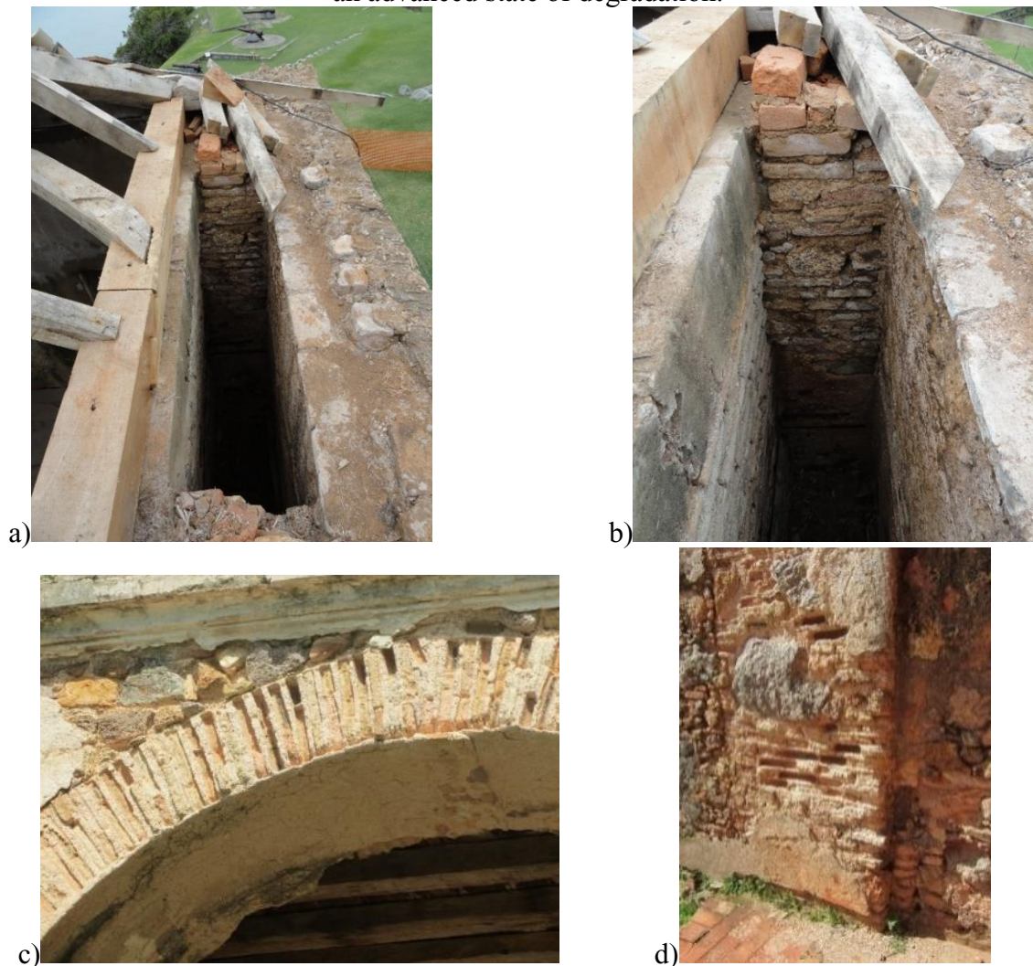
Figure 79 - Stratigraphy of second-level masonry walls (a, b), presence of voids due to the pre-existing chimney. Mortar in good condition in arches (c) and columns (d), while bricks in an advanced state of degradation.
