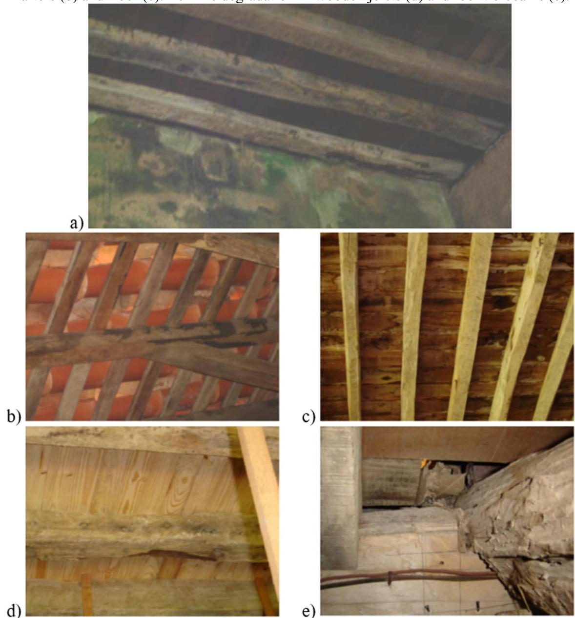
Figure 82 - Advanced degradation of floor joists caused by fungi (a), moisture stains on roof rafters (b) and floor (c). Termite degradation in wooden joists (d) and roof tie-beams (e).
