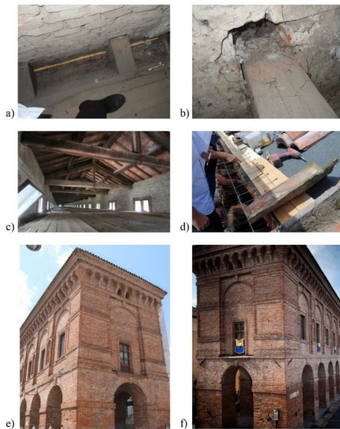
Figure 46 - As-built state after the 2012 earthquake (a, b, c, e) on the structural elements carried out timber joist of lacunar ceiling (a, b), timber roof truss (c, d). Restoration works with steel reinforcement steel tie-rod in masonry walls (f) and modification in the roof extrados (d).
