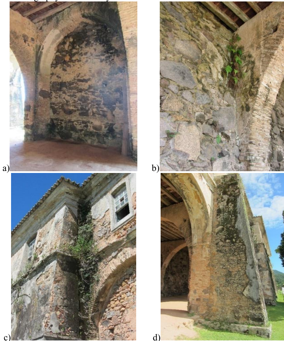
Figure 78 - Stratigraphy of a masonry wall and transversal connection with the retaining wall.
