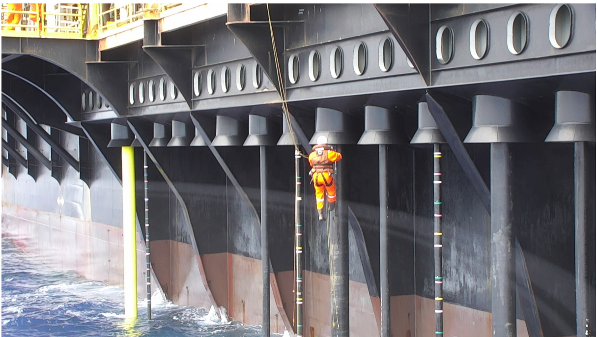
Figure 3 – Technical inspection using industrial climb.
