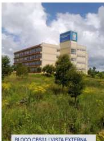
BLOCO CBS01 | VISTA EXTERNA
