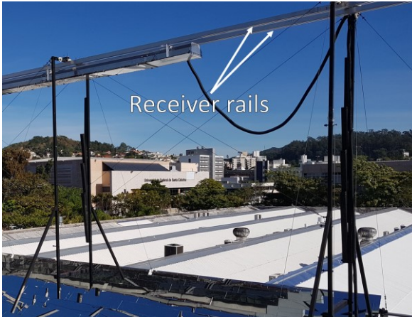
Figure B- 7- Fixation of the receiver on rails.
