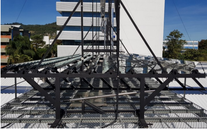
Figure B- 12 - Detailed view of the tracking mechanism on the LFC.
