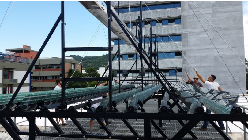
Figure B- 10 - Rising procedure of the receiver.
