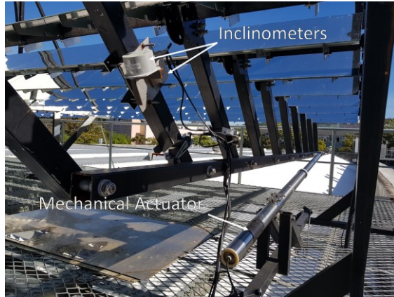
Figure B- 13 - Inclinometers and mechanical actuator installed on the LFC.
