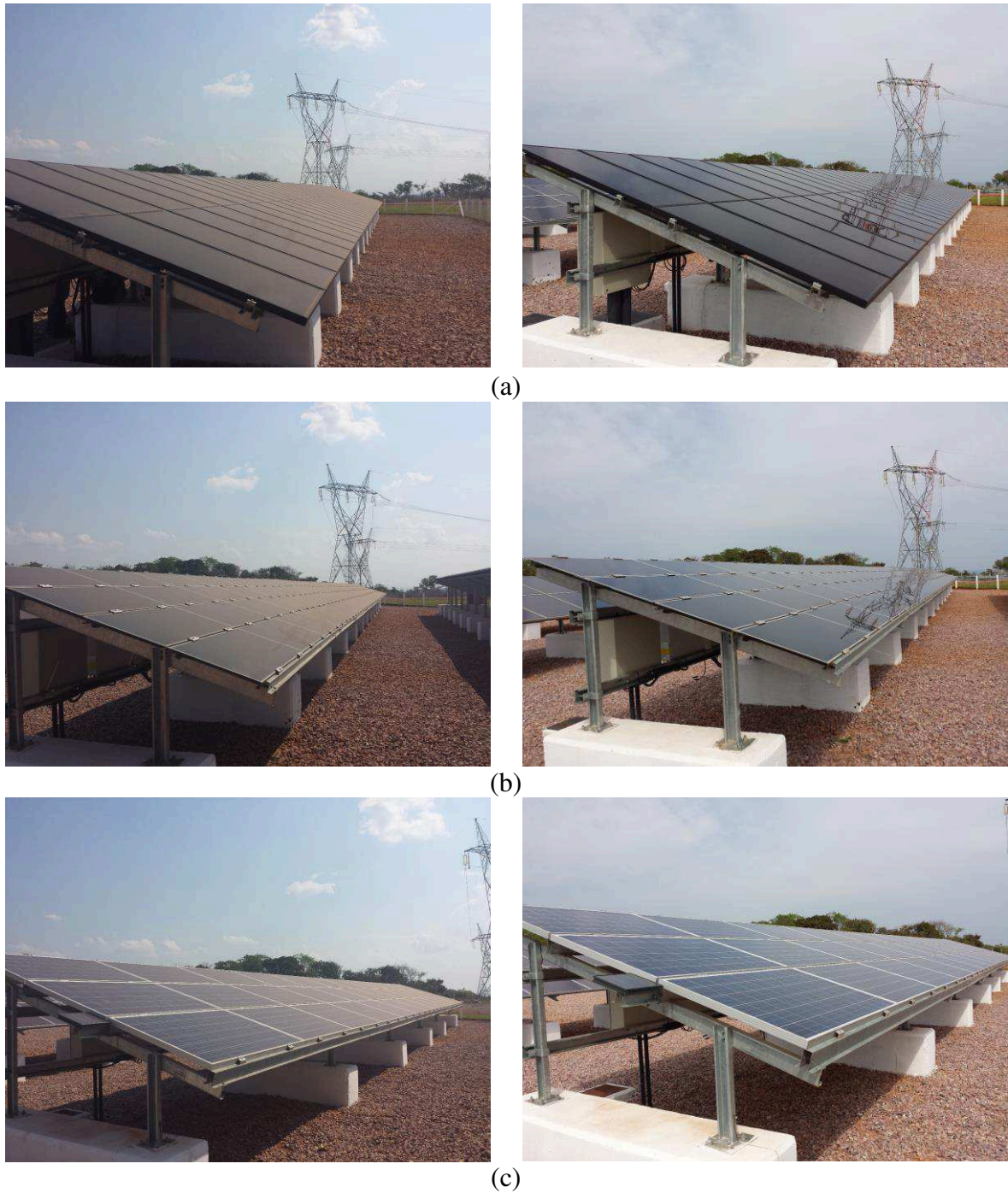
Figure 36 - Images of the CIGS (a), CdTe (b) and m-Si (c) Itiquira MT ES PV systems before and after being manually cleaned (left- and right-hand side images, respectively). The soiling shown was accumulated between December 2013 and September 2014.
