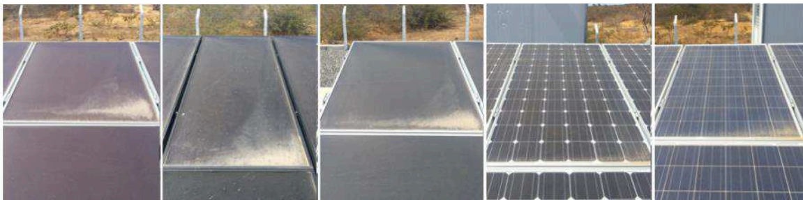
Figure 15 - Non-uniform soiling distribution profile in PV modules caused by high wind incidence (Hickel et al. , 2016).
