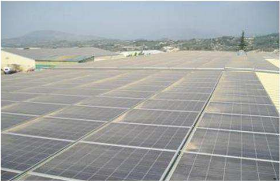
Figure 16 - Non-uniformity of soiling in a PV system (Lorenzo et al. , 2013).
