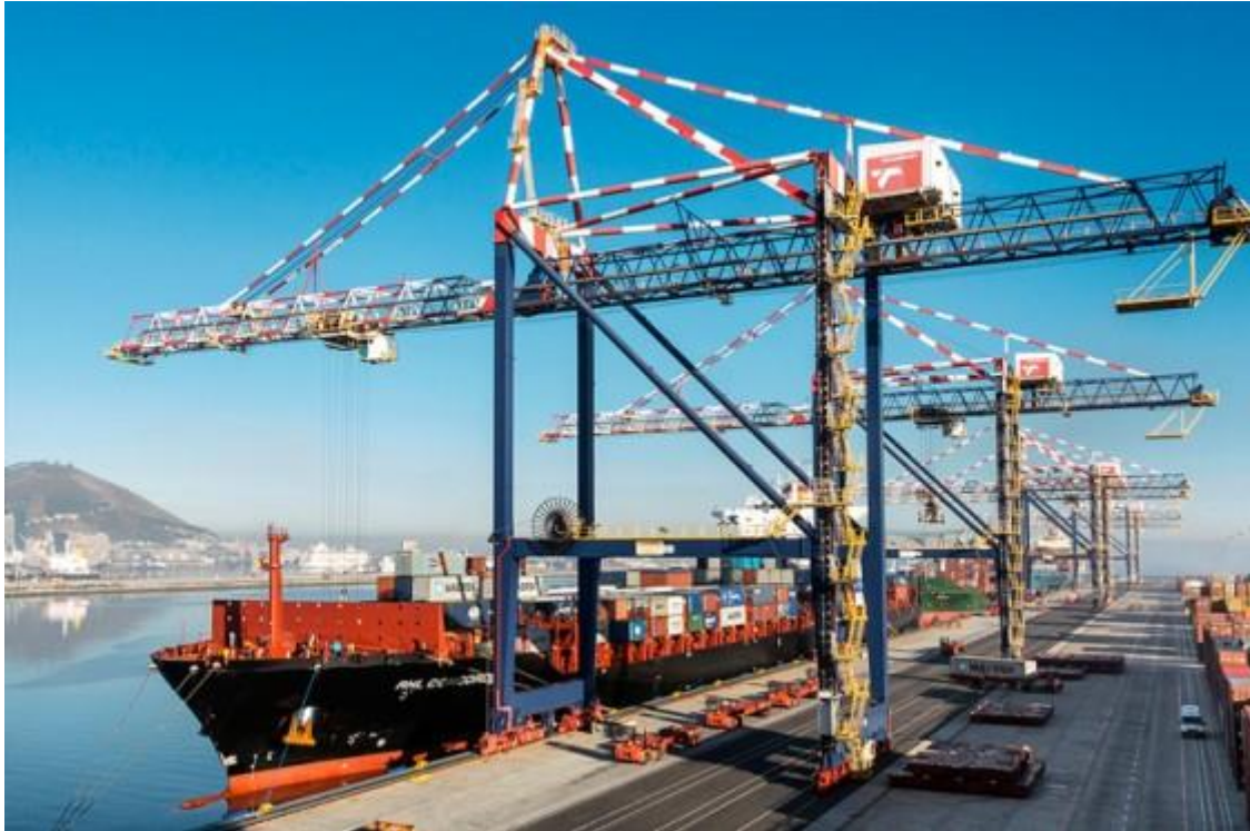
Figura 14 – Ship to Shore Crane (STS)
