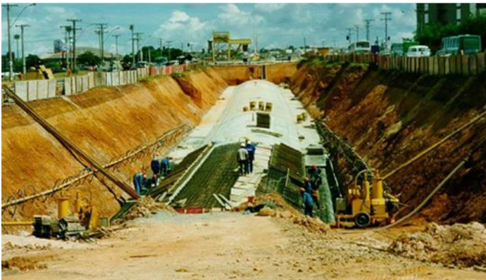
Figura 2.13 – Cut-and-Cover (EARTH MECHANICS, 2016)
