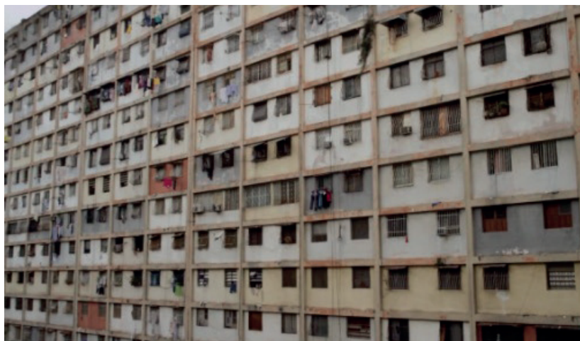
Figure 16: The façade of a building in the housing project.
