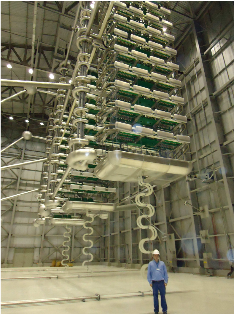
Figura 4.5 – Capacitor Commutated Converter Back-to-Back.
