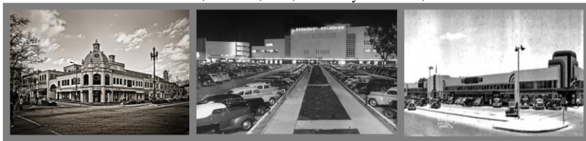
Figura 60 - Country Club Plaza, Kansas, E.U.A. (1923), The Westheimer/Montrose Shopping Center, Houston, 1930, Broadway Crenshaw, 1940
