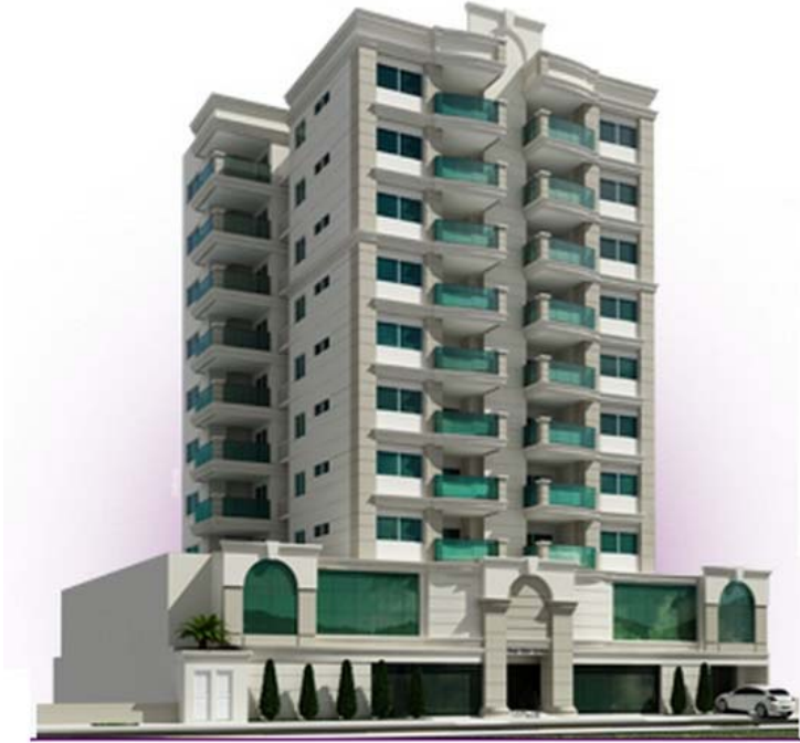
Figura 7 - Fachada Champs Elyseés residence
