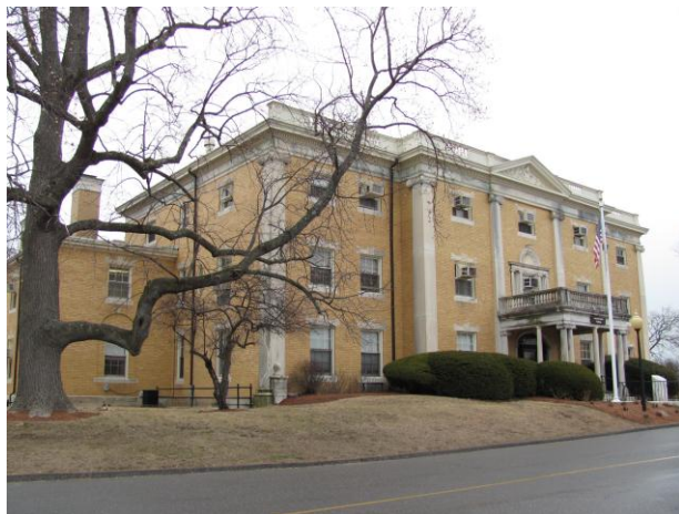
12 McLean Hospital – Administration Building
