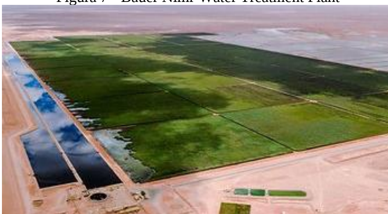
Figura 7 - Bauer Nimr Water Treatment Plant
